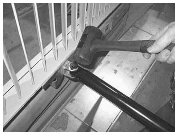
FIGURE 61: DOOR LATERAL ADJUSTMENT
