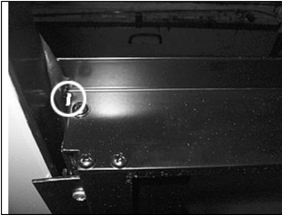
FIGURE 70 : AWNING WINDOW – SEAL THE CHINK
