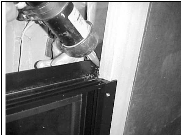
FIGURE 69 : AWNING WINDOW – SEAL THE UPPER CORNERS
