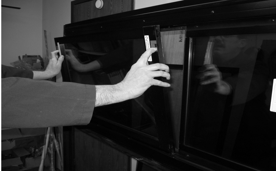
FIGURE 22: REMOVING THE SASH
