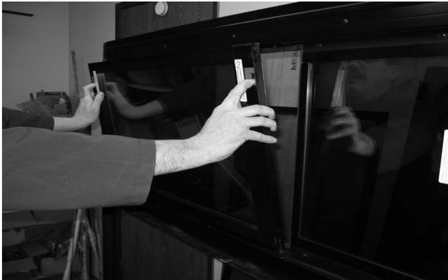
FIGURE 42: REMOVING THE SASH
