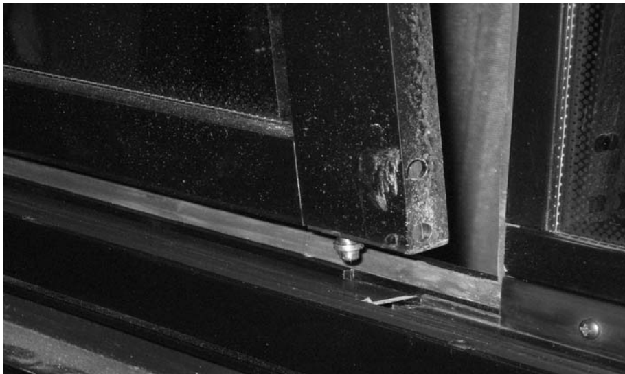
FIGURE 43: DISENGAGING THE BOTTOM OF THE SASH
