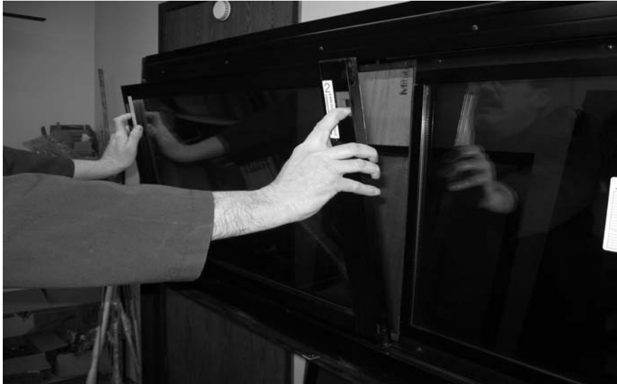
FIGURE 42: REMOVING THE SASH
