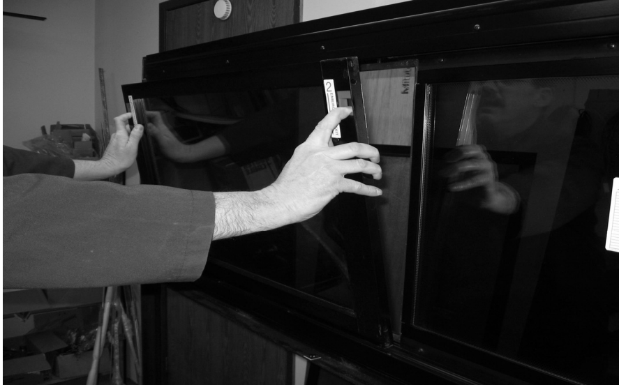
FIGURE 21: REMOVING THE SASH
