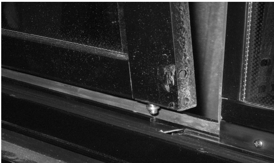
FIGURE 22: DISENGAGING THE BOTTOM OF THE SASH
