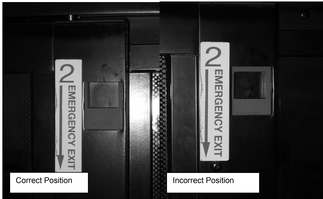
FIGURE 25: RELEASE LATCH PROPER POSITION
