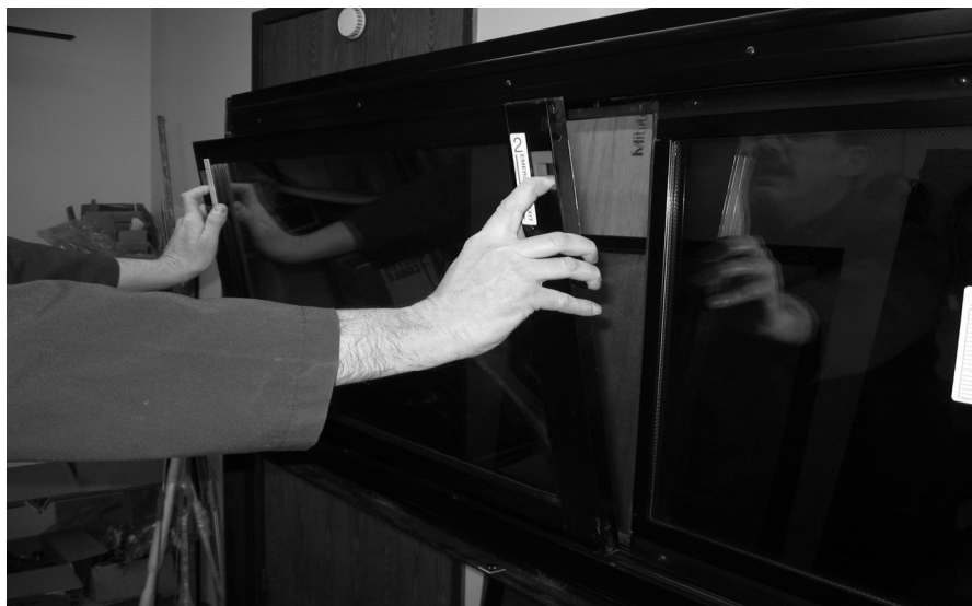
FIGURE 41: REMOVING THE SASH
