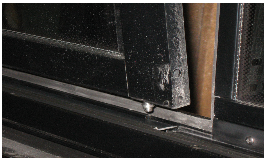
FIGURE 63: DISENGAGING THE BOTTOM OF THE SASH
