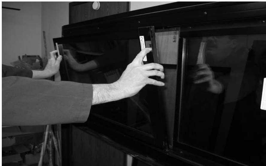
FIGURE 41: REMOVING THE SASH
