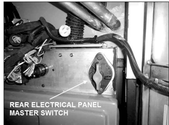
REAR ELECTRICAL PANEL IN R.H. ENGINE COMPARTMENT
