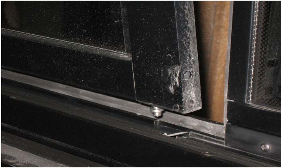
FIGURE 42: DISENGAGING THE BOTTOM OF THE SASH
