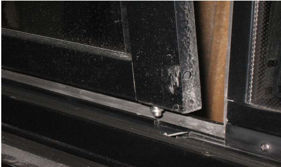
FIGURE 42: DISENGAGING THE BOTTOM OF THE SASH
