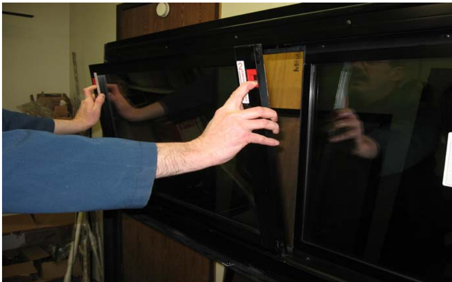
FIGURE 41: REMOVING THE SASH
