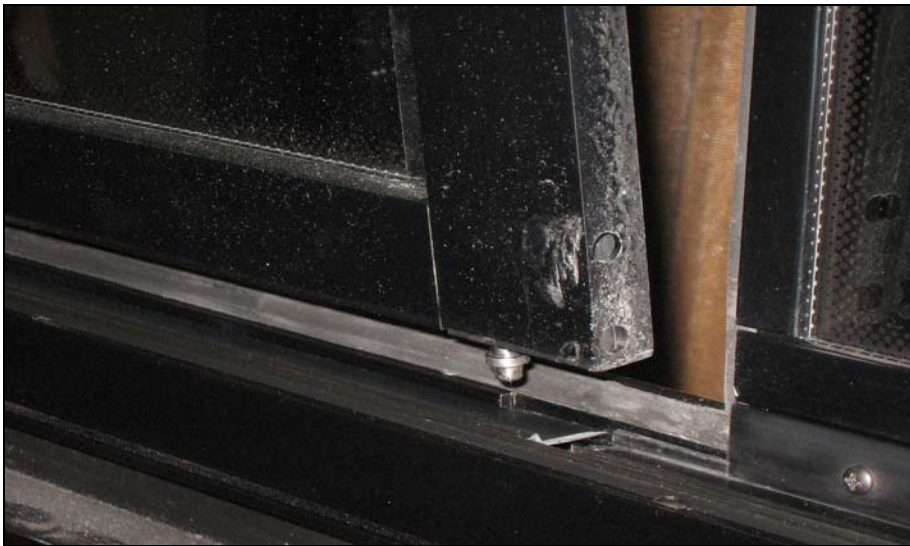
FIGURE 65: DISENGAGING THE BOTTOM OF THE SASH
