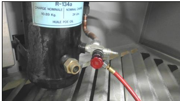
FIGURE 80: RECOVERY UNIT CONNECTED TO RECEIVER SERVICE PORT
