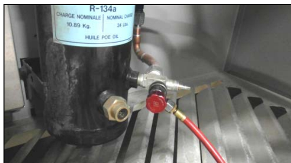
FIGURE 78: RECOVERY UNIT CONNECTED TO RECEIVER SERVICE PORT
