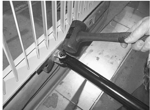
FIGURE 73: DOOR LATERAL ADJUSTMENT
