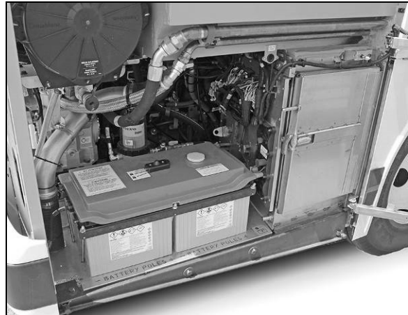
ENGINE COMPARTMENT R.H. SIDE
