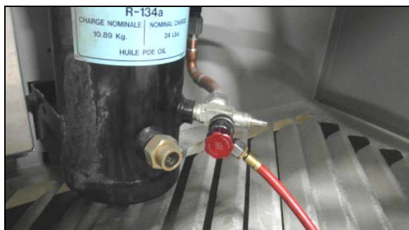
FIGURE 78: RECOVERY UNIT CONNECTED TO RECEIVER SERVICE PORT
