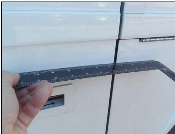
FIGURE 57: USE A RULER (SHOWN IN BLACK) TO CHECK THAT SURFACES ARE EVEN
