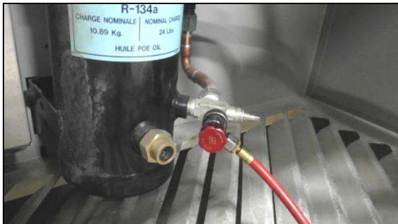
FIGURE 83: RECOVERY UNIT CONNECTED TO RECEIVER SERVICE PORT
