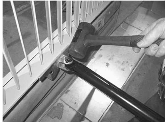
FIGURE 64: DOOR LATERAL ADJUSTMENT
