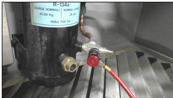
FIGURE 83: RECOVERY UNIT CONNECTED TO RECEIVER SERVICE PORT
