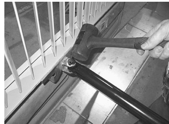
FIGURE 65: DOOR LATERAL ADJUSTMENT
