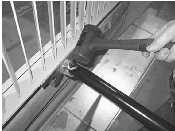
FIGURE 64: DOOR LATERAL ADJUSTMENT
