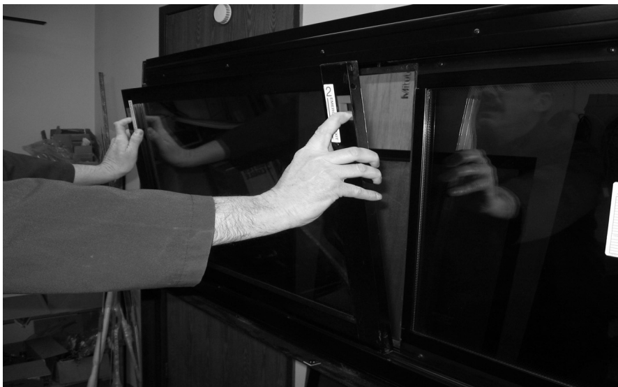
FIGURE 41: REMOVING THE SASH
