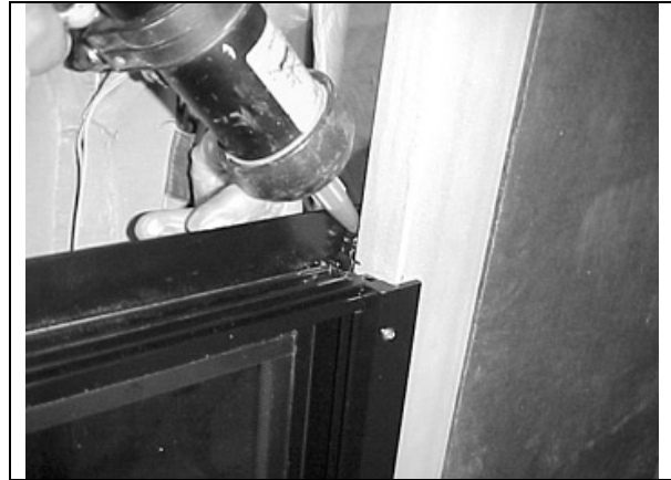
FIGURE 75 : SLIDING WINDOW – SEAL THE UPPER CORNERS
