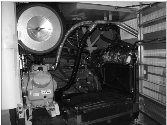
FIGURE 5: REAR ELECTRICAL PANEL, JUNCTION PANEL & BATTERY COMPARTMENT
