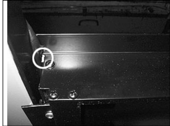
FIGURE 70 : AWNING WINDOW – SEAL THE CHINK
