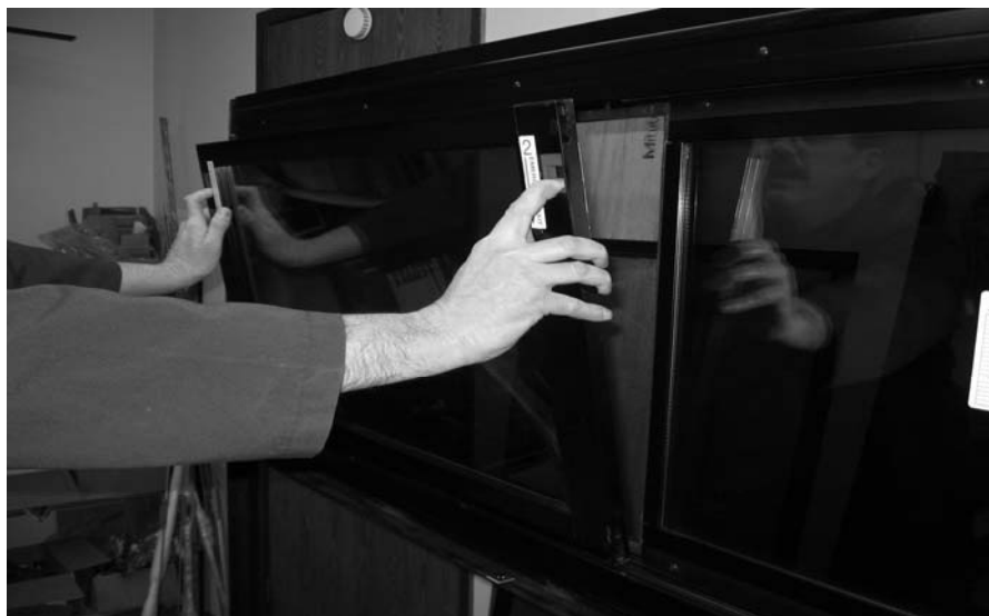
FIGURE 41: REMOVING THE SASH
