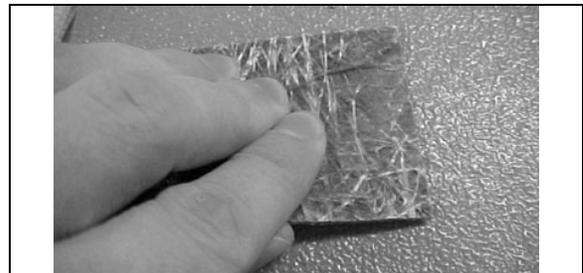
Allow drying for at least **2 hours** then repaint as per paragraph: Minor Repair.
