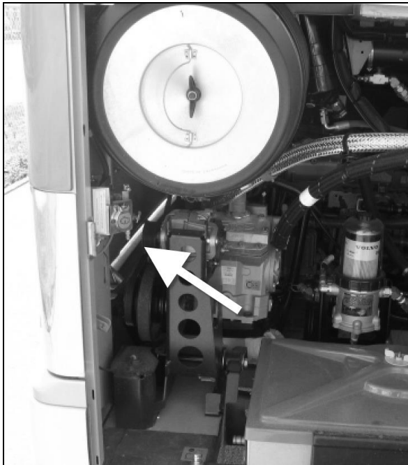
ENGINE COMPARTMENT (TYPICAL)
