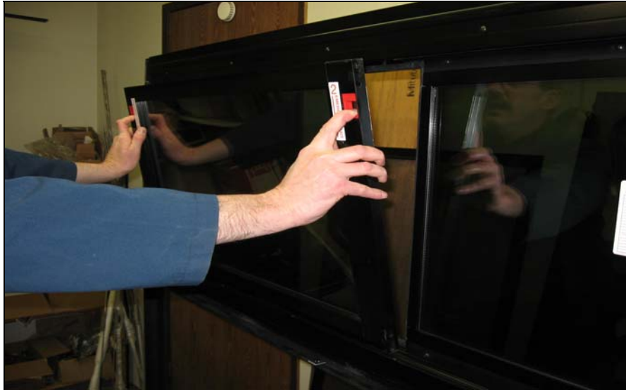
FIGURE 95: REMOVING THE SASH
