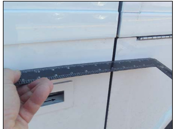
FIGURE 57: USE A RULER (SHOWN IN BLACK) TO CHECK THAT SURFACES ARE EVEN
