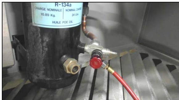
FIGURE 78: RECOVERY UNIT CONNECTED TO RECEIVER SERVICE PORT
