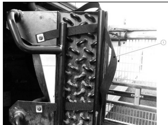
CONDENSER COMPARTMENT STRAP
