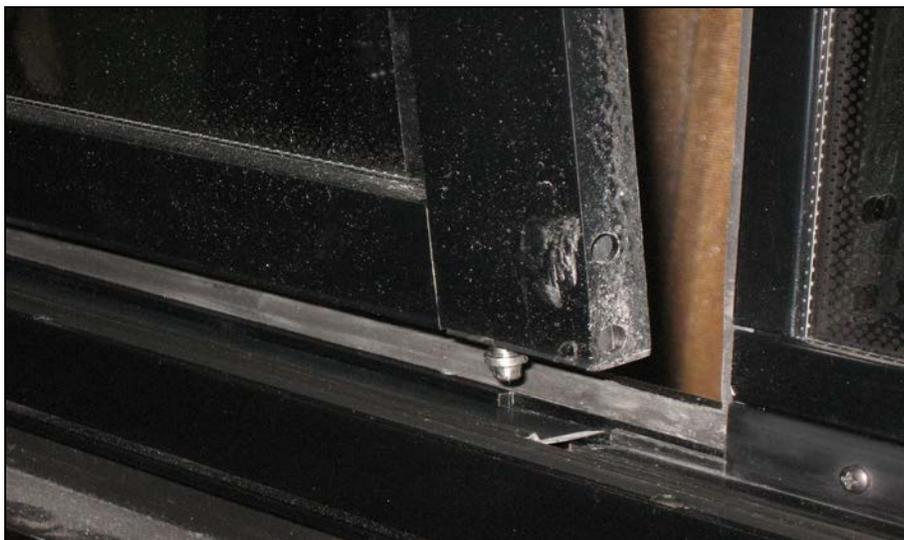
FIGURE 101: DÉGAGEMENT DU BAS DU CHÂSSIS
