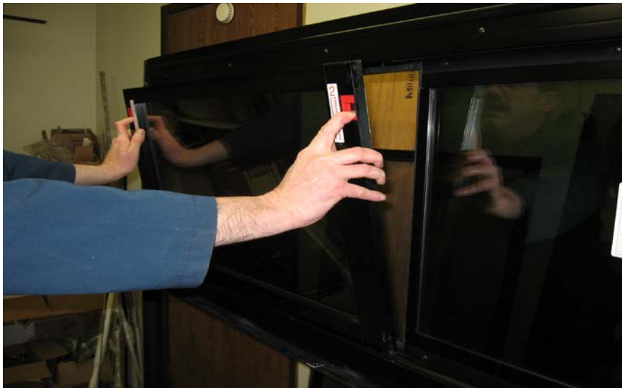
FIGURE 41: REMOVING THE SASH
