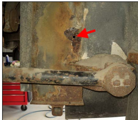
FIGURE 7: HOLE DRILLED IN STRUCTURAL MEMBER
