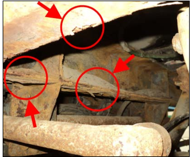
FIGURE 3: METAL FLAKING AND ACCUMULATED SAND
