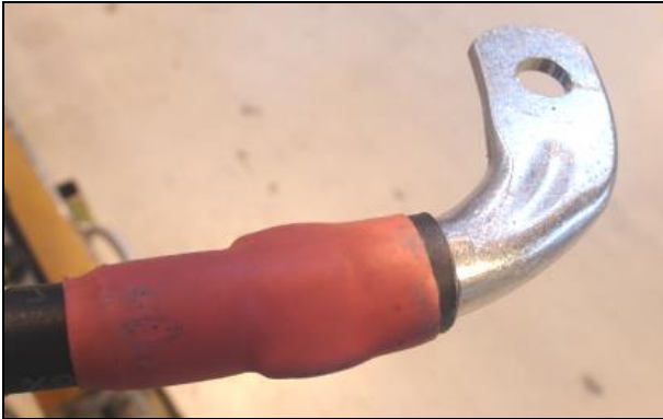
Figure 14: Power cable shouldn't be bent just next to the cable lug. Angled cable lugs are used to avoid mechanical stress.
