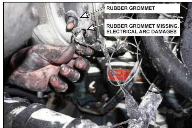
Figure 22: Fire in engine compartment caused by rubbing of power cable against metal edge of Bosch T1 alternator rear cover. Lower rubber grommet was missing when fire occurred. Evidence of electrical arc can be seen.
