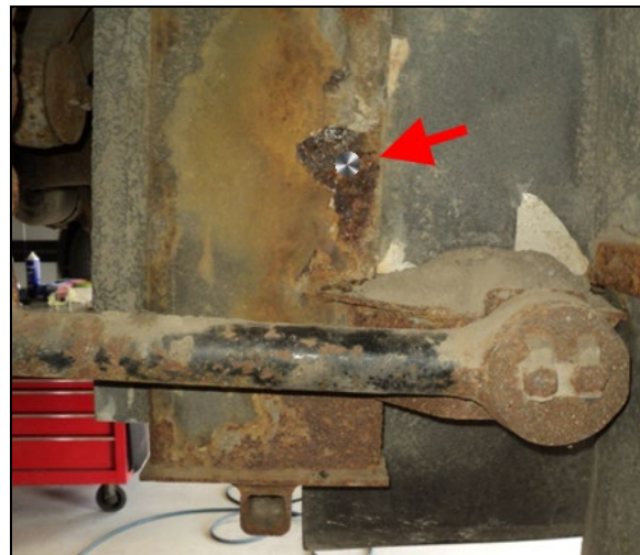
FIGURE 6: CLEANED SPOT ON STRUCTURAL MEMBER
