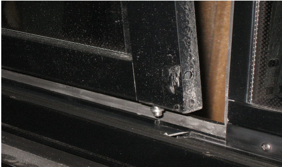
FIGURE 42: DISENGAGING THE BOTTOM OF THE SASH
