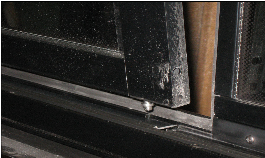
FIGURE 105: DISENGAGING THE BOTTOM OF THE SASH
