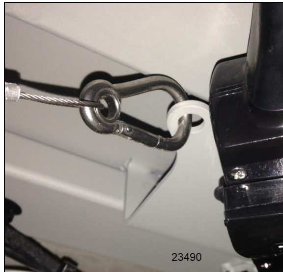
FIGURE 54: PROTECTIVE WIRE INSTALLATION
