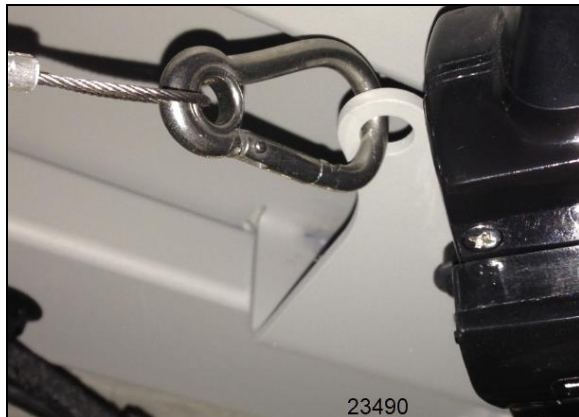
FIGURE 56: PROTECTIVE WIRE INSTALLATION
