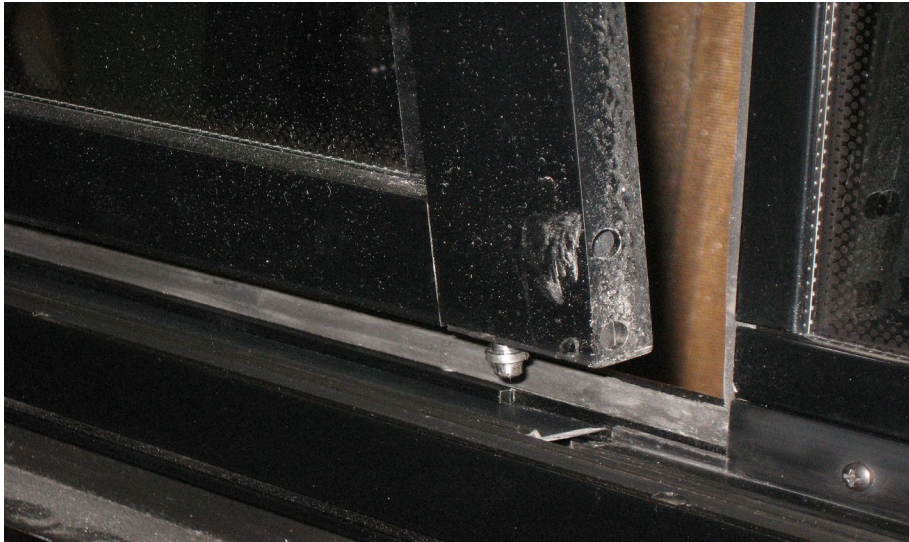
FIGURE 45: DISENGAGING THE BOTTOM OF THE SASH
