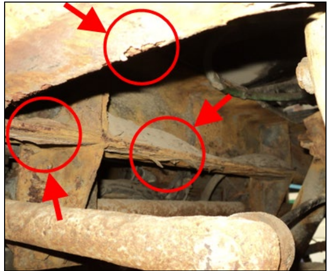
FIGURE 3: METAL FLAKING AND ACCUMULATED SAND
