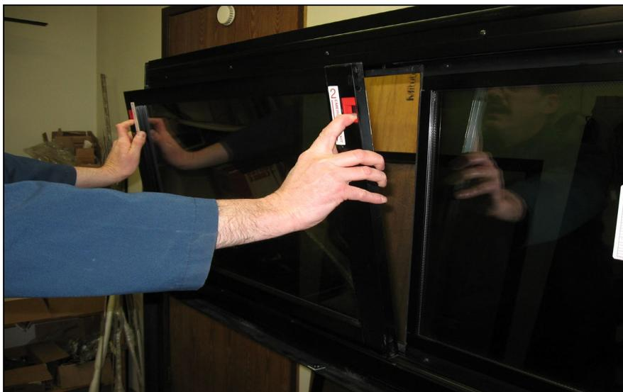
FIGURE 103: RETRAIT DU CHÂSSIS
