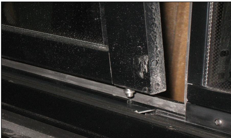
FIGURE 104: DÉGAGEMENT DU BAS DU CHÂSSIS
