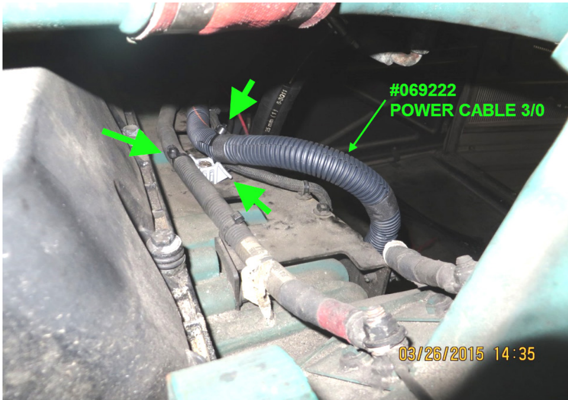
FIGURE 14: POWER CABLE ATTACHED TO #2 DOUBLE-TIE MOUNT AND PROPER NYLON TIES INSTALLATION
