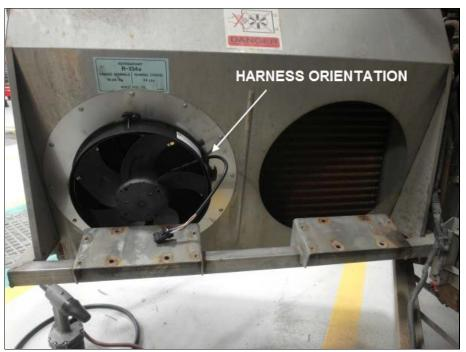
11. Use the remaining ring as a template to position the upper (exterior) fan. Center the ring on the upper part of the shroud, from left to right (horizontally), the center of the ring should match the center of the bottom fan. Up and down (vertically), the lower edge of the ring must not be installed more than 20mm from the lower edge of the fan shroud as seen in the picture below. Using a sharpie or a sharp pointed tool, draw the opening position on the top part of the shroud.
