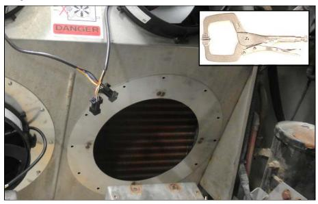
25. Drill the ring top, bottom and side rivet holes (4X) & secure the ring to the shroud using supplied rivets (remove C-clamps pliers).
