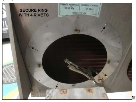
9. Drill the remaining rivet holes around the adaptor ring perimeter and install rivets to finalize the ring installation.
