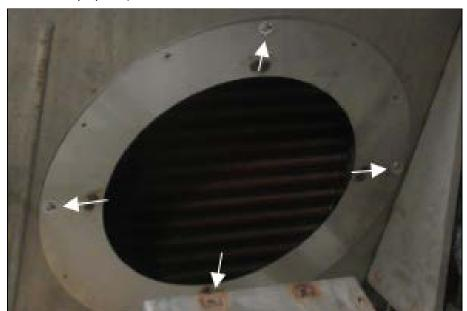
26. Drill the remaining rivet holes around the adaptor ring perimeter & install the last rivets to finalize the ring installation.
