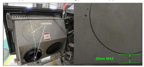
12. Using a high speed cutting tool, cut the upper fan opening.
