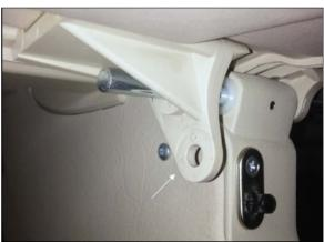
4. Unlock the door pivot rod using a 2mm hex key (Allen wrench).
