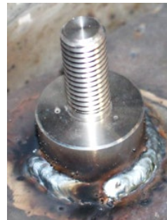
FIGURE 79: GROUND STUD #380360
