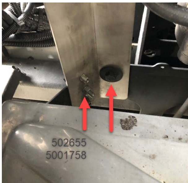
FIGURE 31: INSTALLATION DU PILIER SUPPORT
