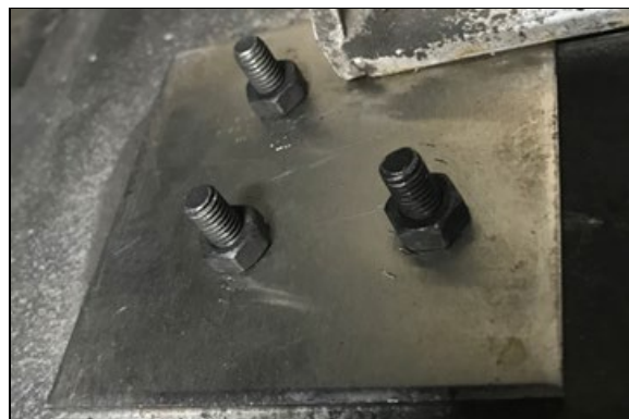
FIGURE 22: PLAQUE DE RENFORT INSTALLÉE
