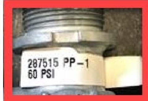
Figure 2: PUSH-PULL PP-1 TYPE VALVE LABEL
