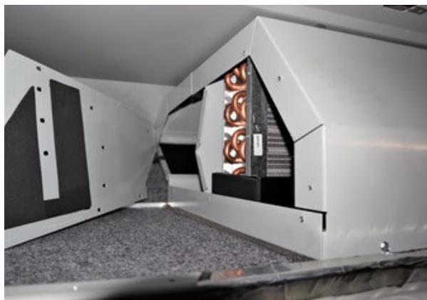
5. Remove cover on the other side of the AC unit (two pieces cover).
