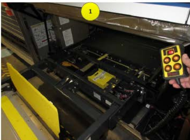
Power up lift, and electrically deploy lift to the outmost position. Turn off power to the lift once complete.
