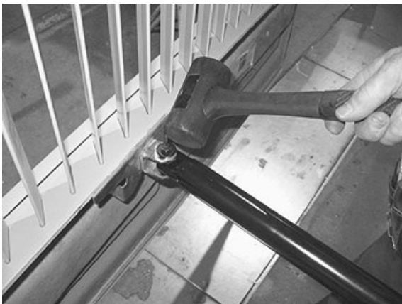
FIGURE 85: DOOR LATERAL ADJUSTMENT
