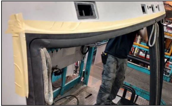
FIGURE 63: MASKING TAPE APPLICATION
