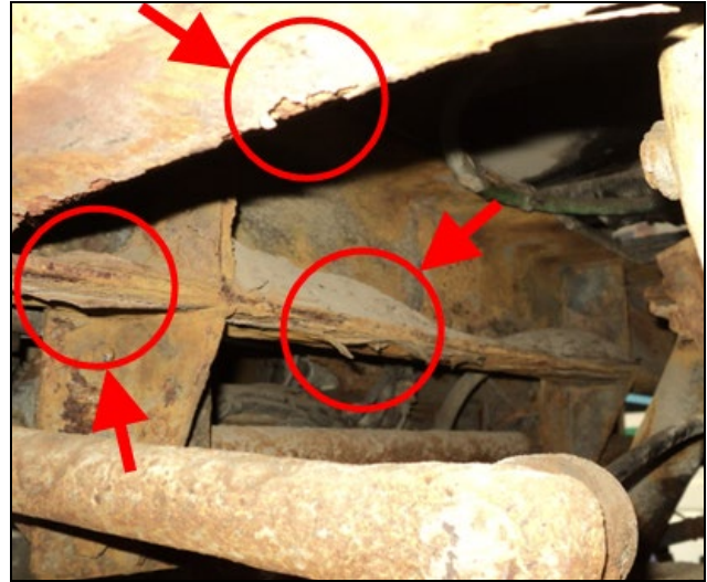
FIGURE 3: METAL FLAKING AND ACCUMULATED SAND
