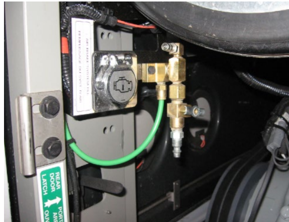
FIGURE 23 : ENGINE COMPARTMENT EMERGENCY AIR-FILL VALVE
