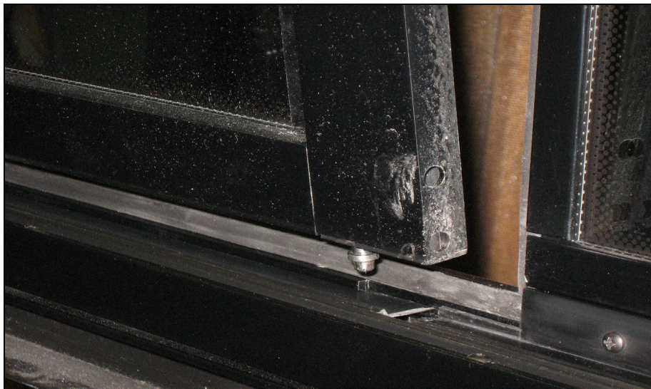
FIGURE 109: DISENGAGING THE BOTTOM OF THE SASH
