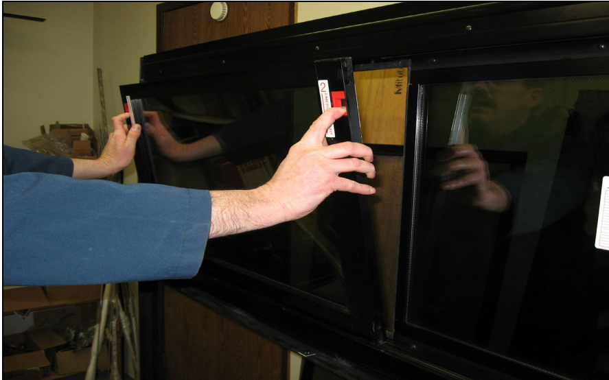
FIGURE 108: REMOVING THE SASH
