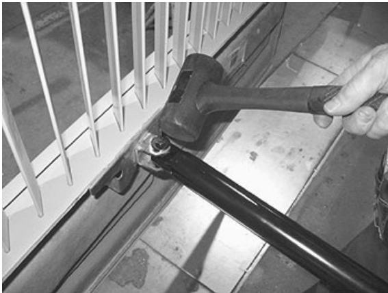
FIGURE 85: DOOR LATERAL ADJUSTMENT
