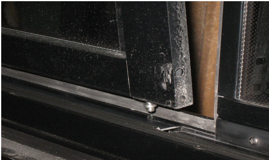
FIGURE 48: DISENGAGING THE BOTTOM OF THE SASH
