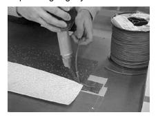
8. The heel of the fast nozzle must not lean against "Tarabus" covering (always parallel to the surface).
