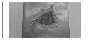
Using a plastic spatula, apply some Sika 221 grey onto the damaged area.
