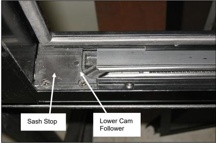
FIGURE 110: PROPER ALIGNMENT
