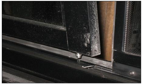
FIGURE 109: DISENGAGING THE BOTTOM OF THE SASH
