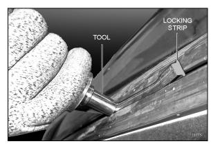
11. IMPORTANT: Every 6 inches or so, slide backwards to compress the strip due to its tendency to contract during drying process.
