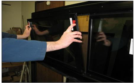
FIGURE 108: REMOVING THE SASH
