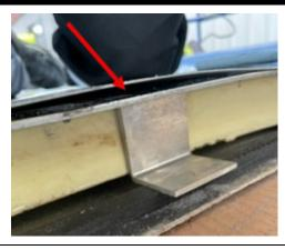
2. Apply glue 684685 between roof panel and structure.
