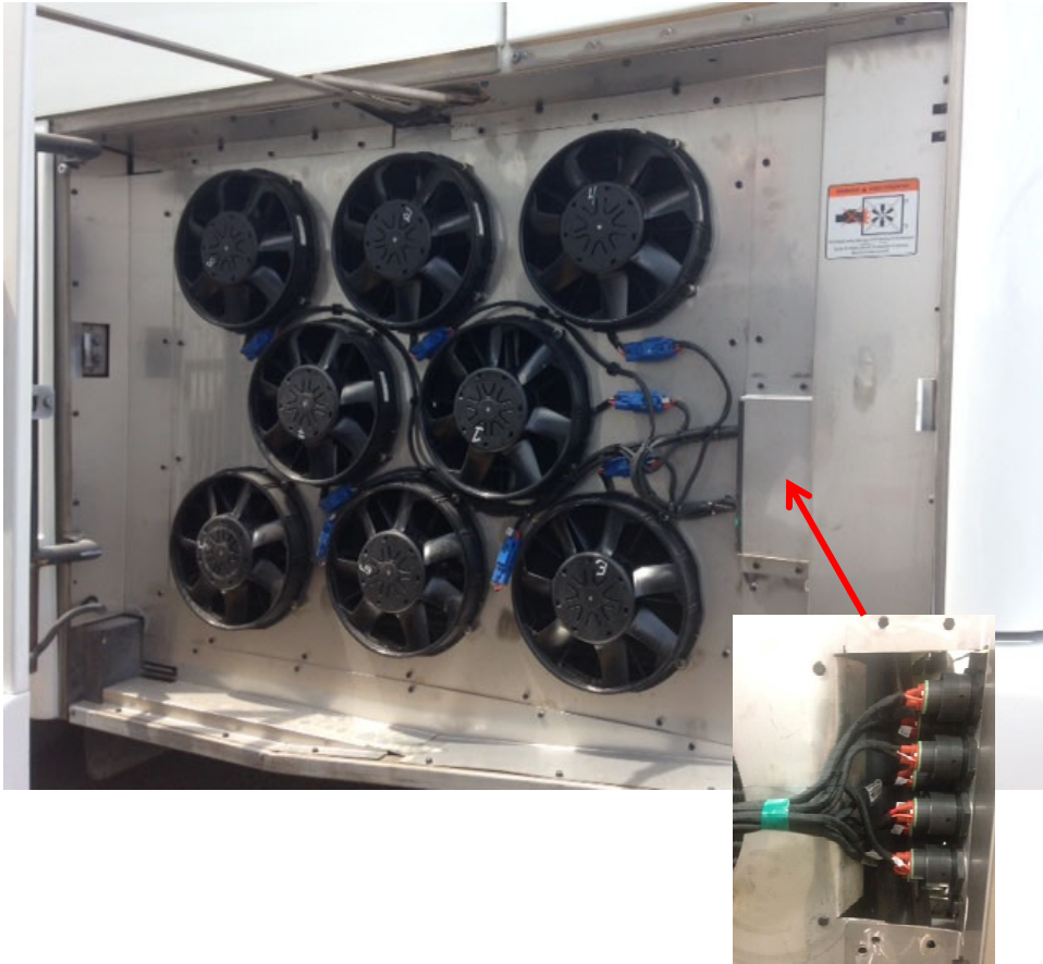
Fan and shroud installation
